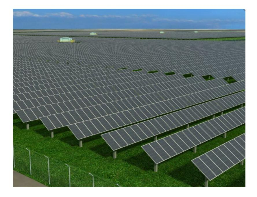
The solar farm will utilize a single-axis tracking system, which enables the solar panels to follow the path of the sun to maximize energy generation. By applying single-axis tracking systems, electricity generation from each solar panel generally increases by 15-25%.
