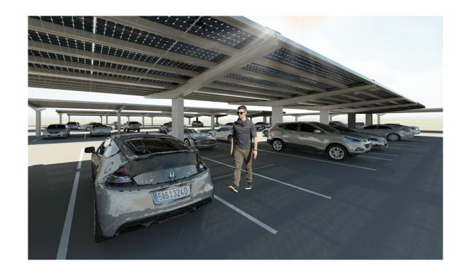
Solar canopy: In addition to generating electricity from the sun, these structures provide shade during summer and protection from precipitation.
