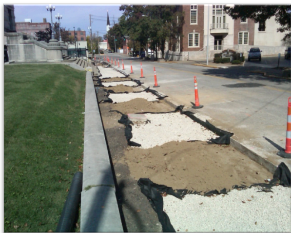
Open graded stone being installed around the Old Courthouse
